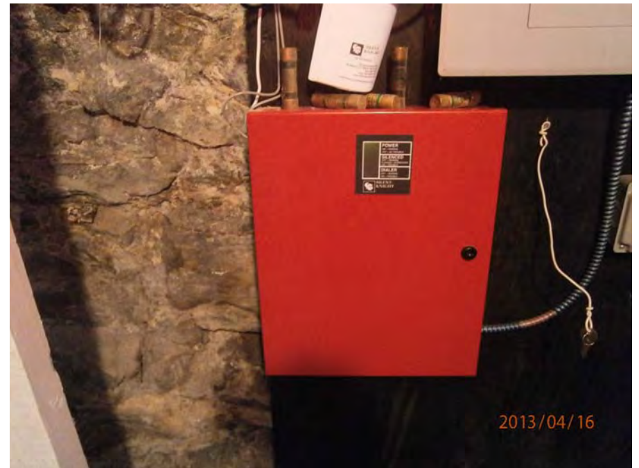
16. Zoned fire control panel
